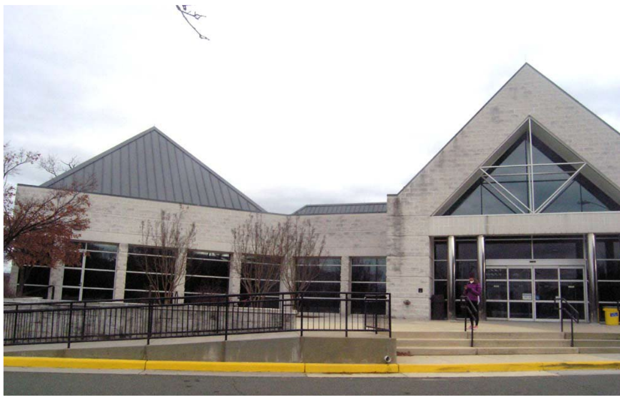
The library building with the event space on the left.
